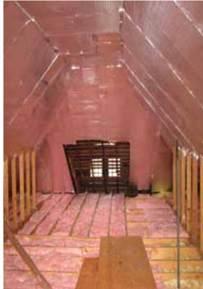
A roof mounted radiant barrier installation in an older home.
